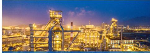
A night view of FHS's twin blast furnaces in Vietnam, which represent China's first export of large-sized ironmaking equipment. They each have a volume of 4,350 cubic metres and were built by CISDI to an EPC mode
