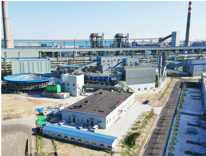
Waste to energy facilities at Shougang Jingtang Steel
