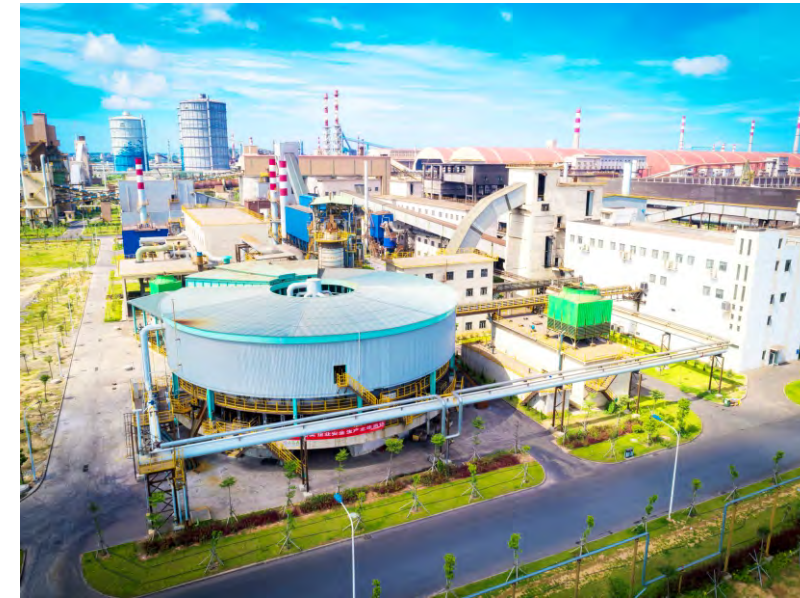
The solid waste centralised treatment centre helping to create a greener Baosteel Zhanjiang
